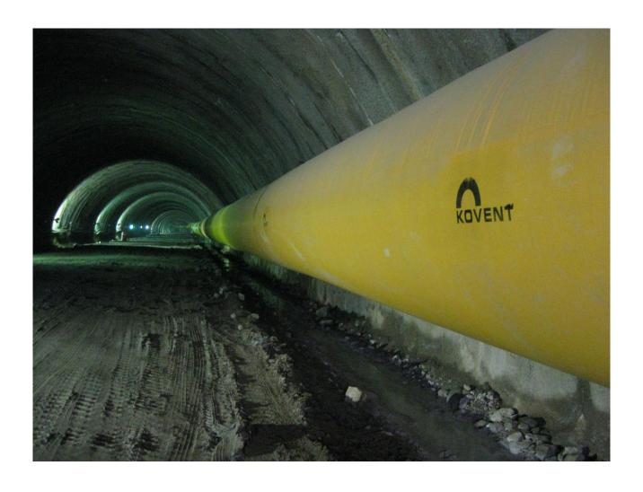
**KITEX FLEXIBLE DUCTING** is manufactured from PVC Coated Polyester Fabric and is distinguished by the relatively low weight with kept high strength values which results in a very pliable and easy to handle duct.
